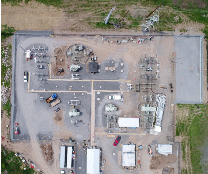
Station 418 – Substation to be expanded and upgraded to accommodate the receipt of Line 949.
