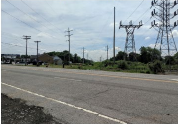
Existing ROW looking southeast from Buffalo Road along proposed improvements, taken July 18, 2019.
